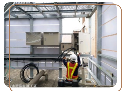
Construction photo taken on 2020.11.12.
