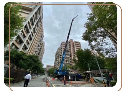
Project construction began on 2020.10.5. Cranes hoisted materials to the site on 2020.10.6.
