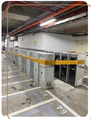
Water dispenser replacement at Blocks A and B of Prince House Changxing.
