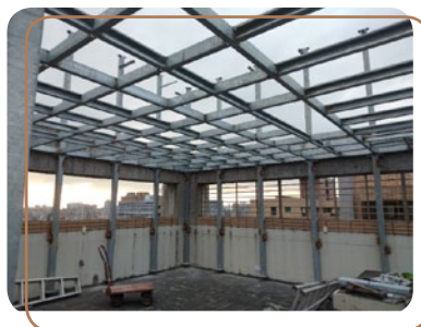
Construction photo taken on 2020.10.28.
