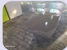
Floor leveling and renewal works of Shuiyuan Lounge - "self-leveling clay work"
